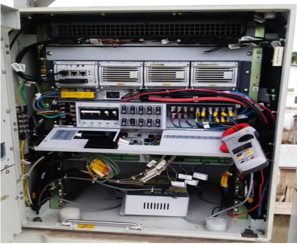
Fig. 5. DC current measurement setup
